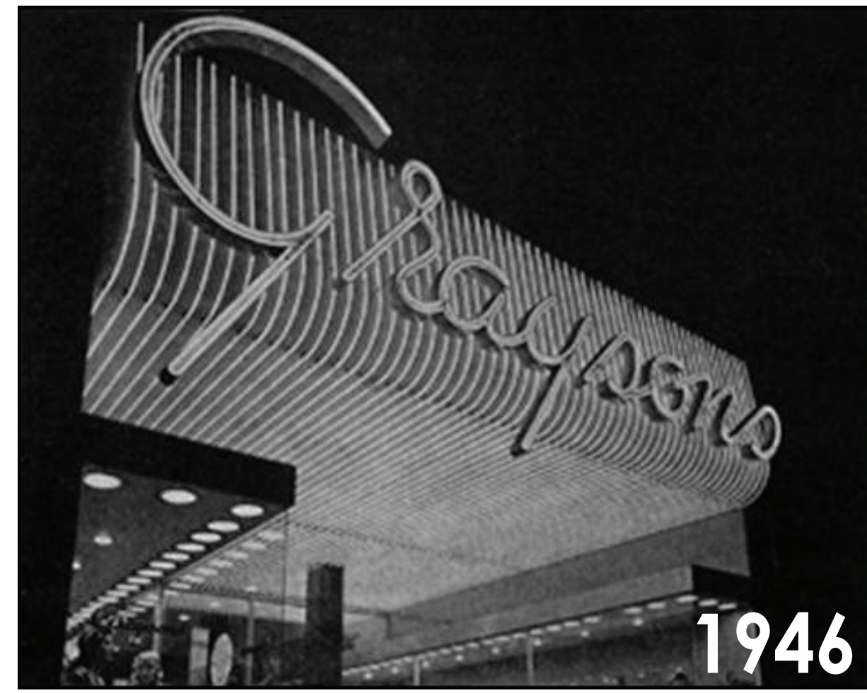
NORTH ELEVATION, DETAIL OF GRAYSON'S STOREFRONT AT NIGHT. LA FORUM ISSUE 7, ORIGINAL SOURCE UNKNOWN | HISTORIC CA. 1946
